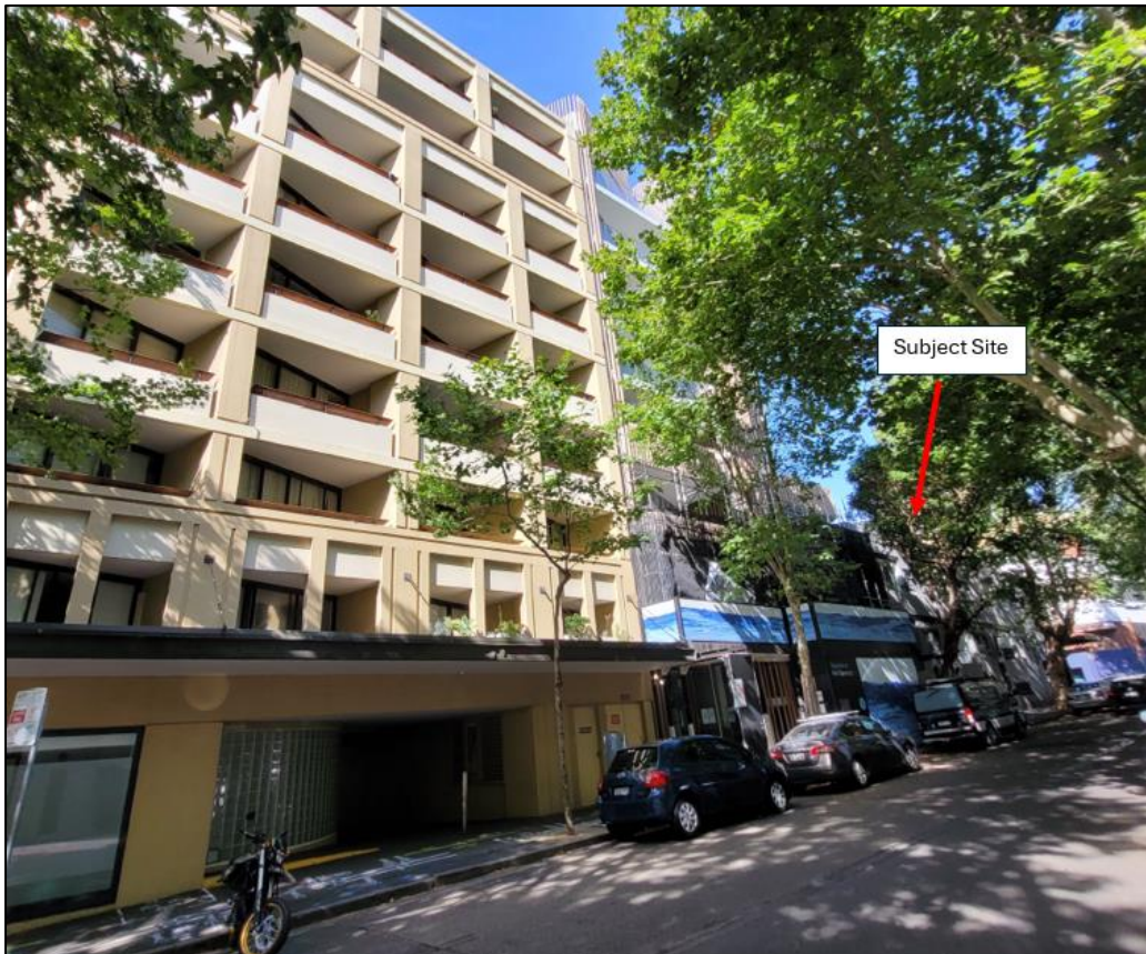
Figure 4: Site viewed from Cooper Street looking north-east
